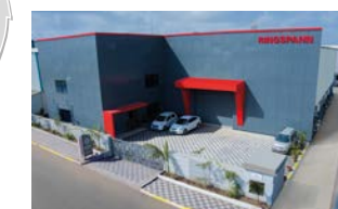
RINGSPANN Power Transmission India Pvt. Ltd., Inde
